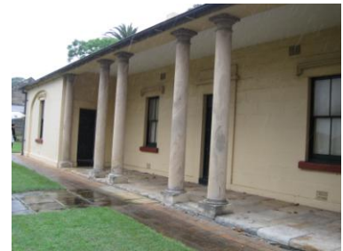
The Barracks - note the rare rounded sandstone pillars made from one piece of sandstone and shaped by hand
