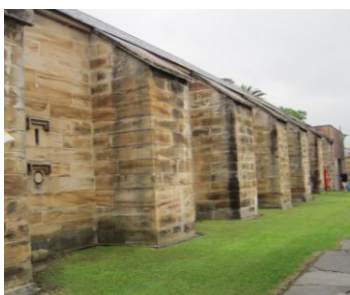
Powder Magazine Wall 2 to 3 meters thick
