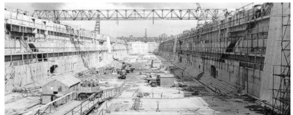
Captain Cook Graving Dry Dock under construction.
